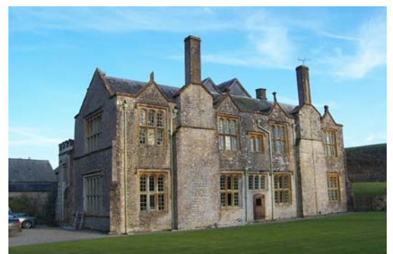
Whitestaunton Manor Major repairs and alterations to Grade I listed medieval manor house
